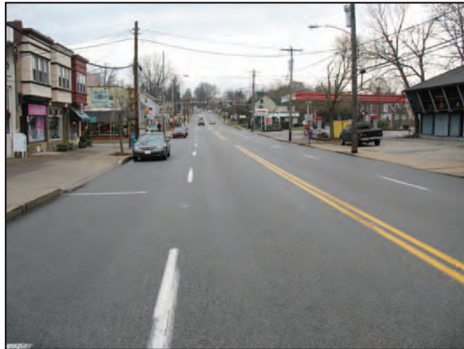
The need for on-street parking and the lack of dedicated parking lanes results in this unusual allowance of on-street parking in an active travel lane — a potentially dangerous condition. (Photo: DVRPC)
