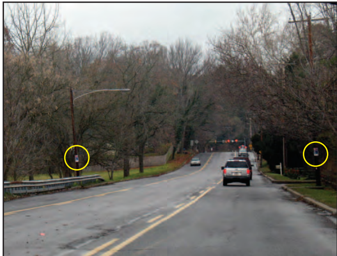
Some areas of the corridor, like this segment just south of Church Road, contain transit stops, but no shelters or safe places to wait. At some points, like the area shown, there are no sidewalks leading to the stops (bus stops are circled in yellow). (Photo: DVRPC)
